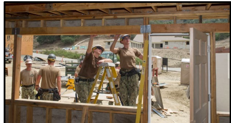
Seabees build "search city" for training center in Santa Paula, CA
