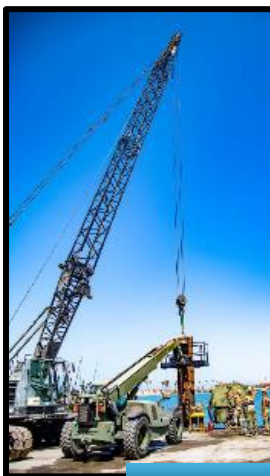
Underwater / Waterfront Construction
