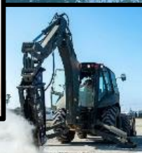
Port and Airfield Repair & Opening
