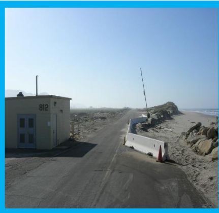
Flooded airfield lights utility bldg- East bound lane gone
